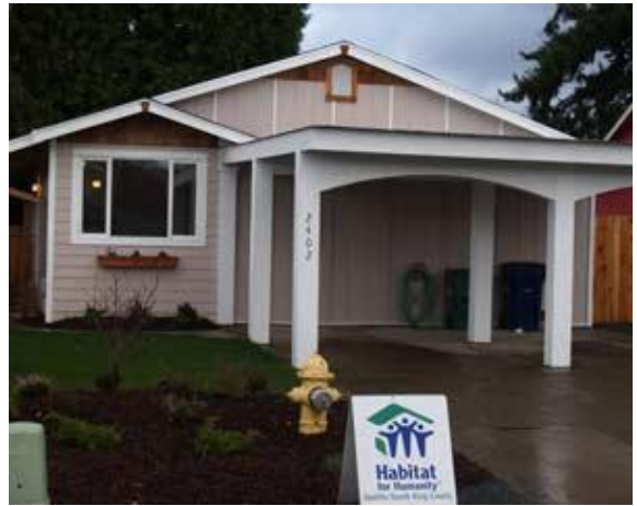
22 Westway home rehabilitation project
