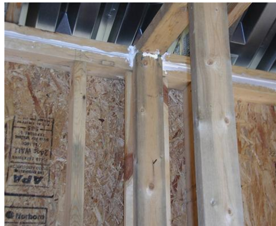
6 24" on center framing and sealed penetrations--TriState
